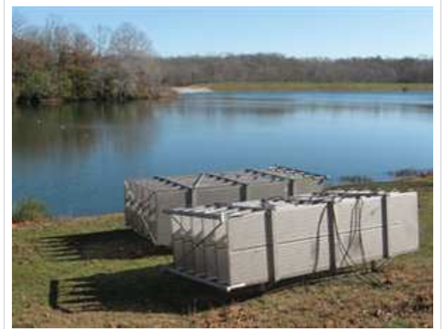
GREEN WORK: Memphis-based engineering firm Allen & Hoshall has seen an increase in energy audits, including the Davy Crockett Park Energy Conservation Project in Lawrenceburg, Tenn. The firm recommended a geothermal lake heat exchange for the park. – PHOTO COURTESY OF ALLEN & HOSHALL
