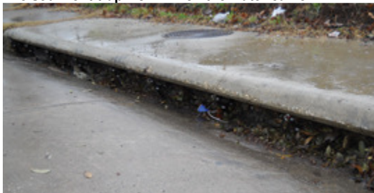
Photo: TERRADYNE GROUP The Curb Companion is seen here in action, trapping leaves and trash.
