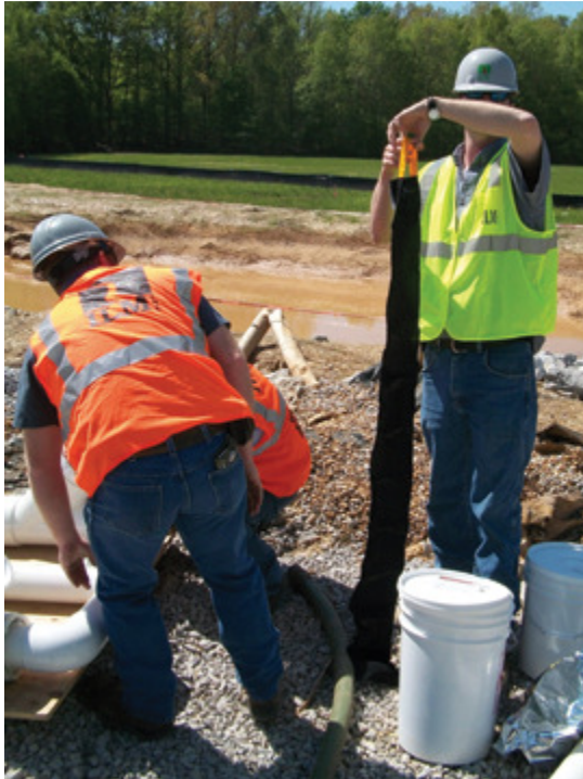
Photo: STORMKLEAR Treatment socks are installed.
